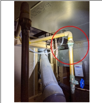
Corrosion/leak of cold water supply
