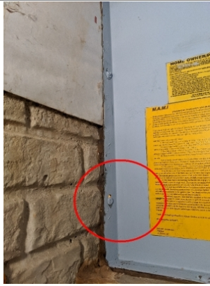
No apparent sealant. Seal to prevent water entering
