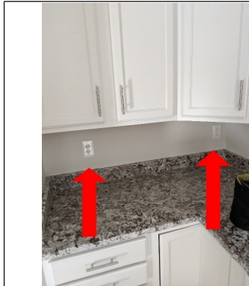
Kitchen counter outlets not GFCI
