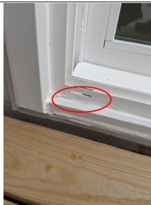
Weep hole has been caulked over
