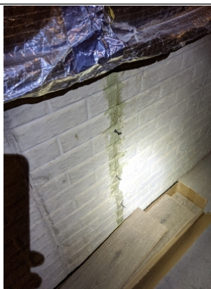
Injection repair of foundation example
