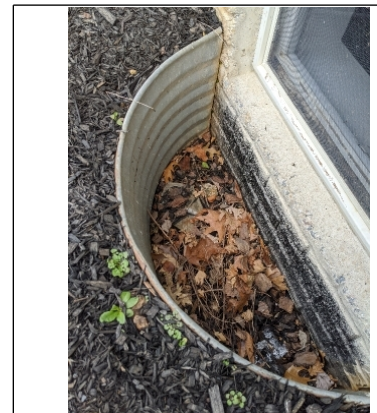
Debris entering window well
