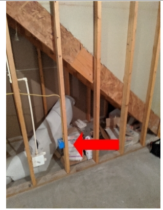
Outlet missing cover plate
