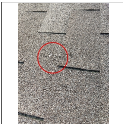
Blistering, typical for shingles at end of useful life
