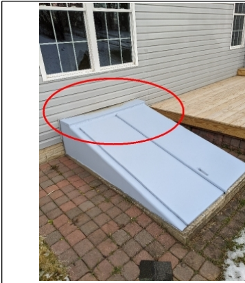
Water accumulation on top of Bilco step cover
