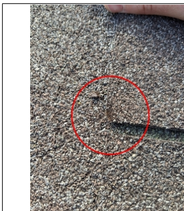
Shingles are brittle due to temp and age
