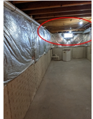
No insulation in cantilever joists under eat-in kitchen
