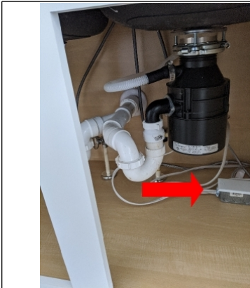
Junction box base of kitchen sink cabinet
