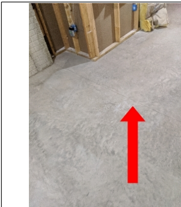
Crack in basement floor
