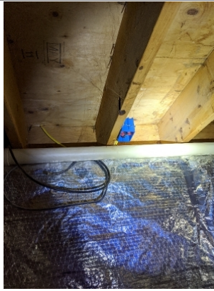
Junction box missing cover plate
