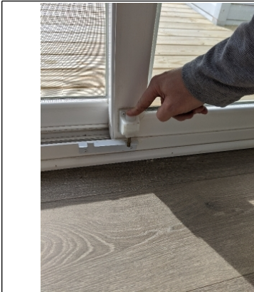
Lock mechanism would not engage on sliding door
