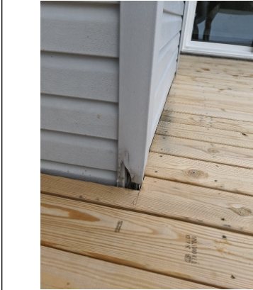
Damage to corner trim at deck
