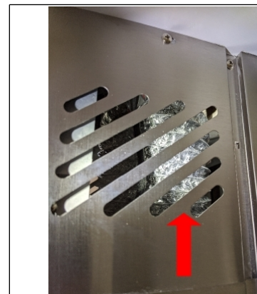
Foil flex duct installed in hood vent
