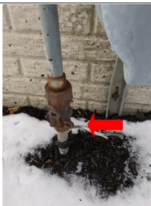
Main gas shut-off on exterior at gas meter
