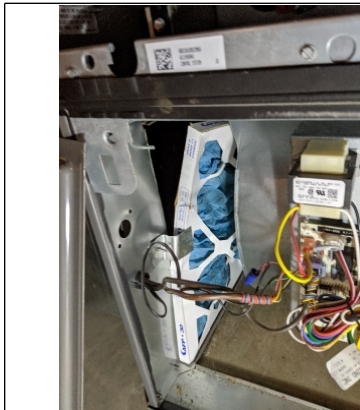
Air filter replacement obstructed and in blower service section of furnace
