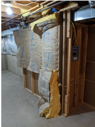
Exposed insulation in unfinished basement area
